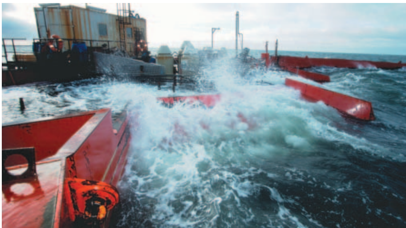
Wave overtopping on the Wave Dragon device [Courtesy: Wave Dragon. Photo: Earth-vision.biz]
