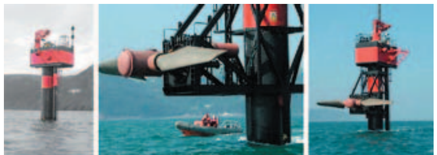
'Seaflow' tidal current turbine [Courtesy of Marine Current Turbines].
